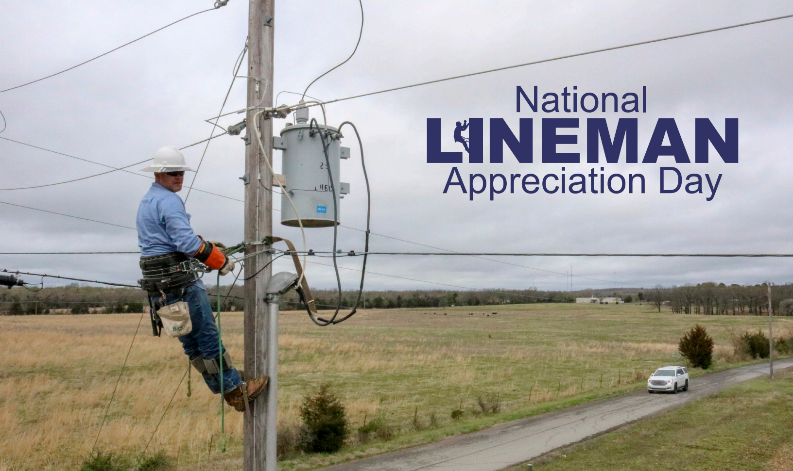
Brad Farrar, LREC Apprentice Lineman, working on members' service line.
