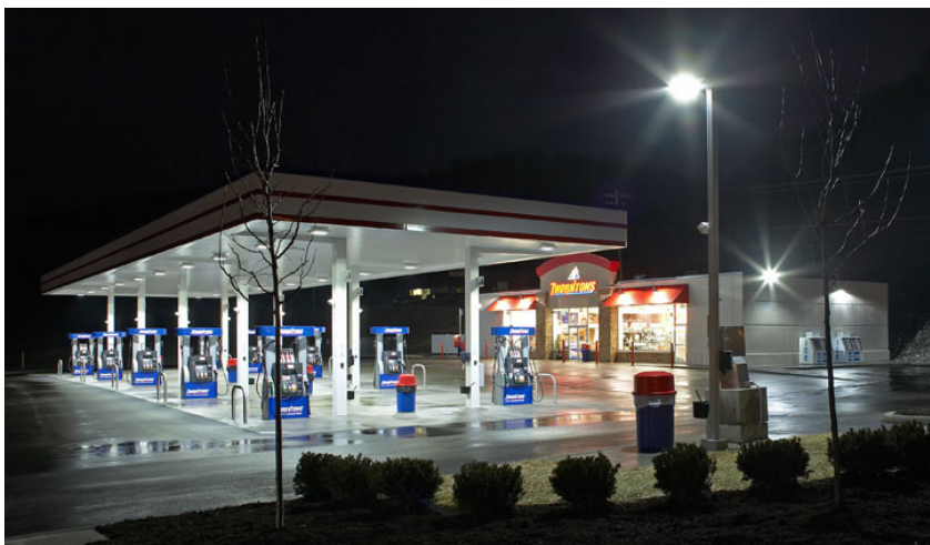
Example of HID parking lot lights
