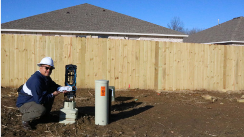
Noe Degollado, LRTC tech, working in Gibson Grove fiber pedestal.
